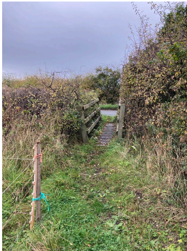
Figure 13: Existing footbridge across ditch at southern crossing location, Wheldrake Lane, Sustrans 2022
